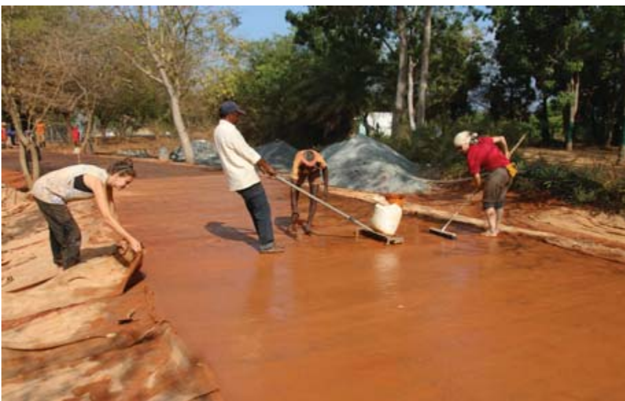
Raking the wearing course to create an abrasive finish
