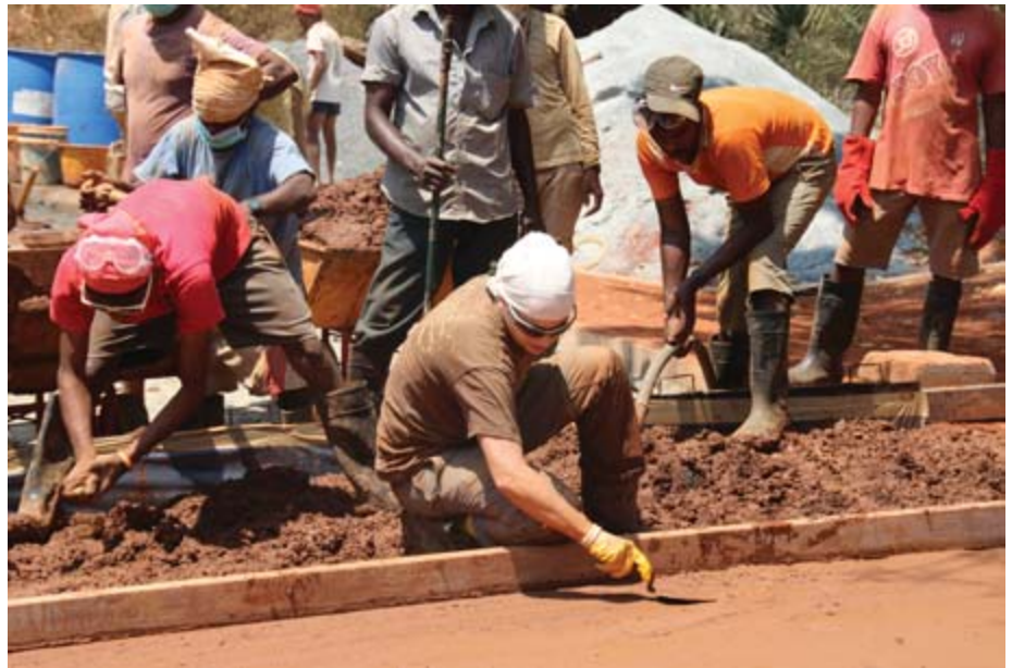
Filling gaps in the wearing course
