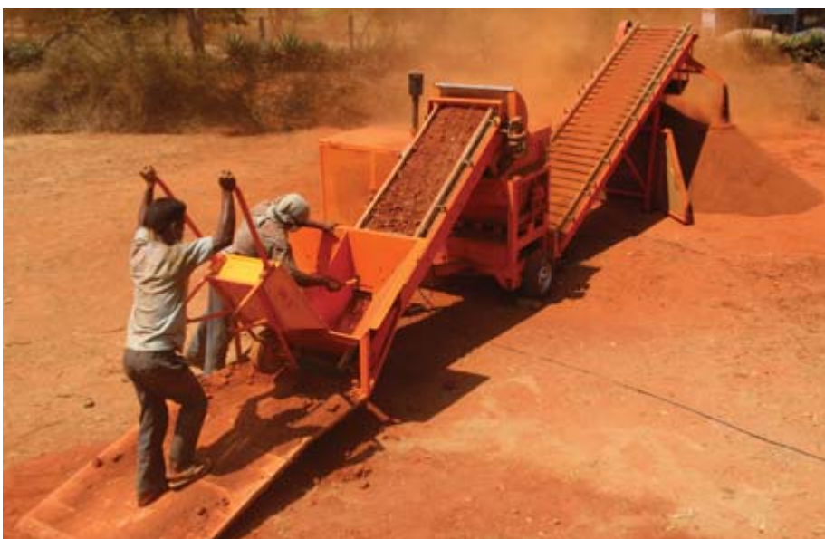
Filling the hopper and breaking up very large clumps
