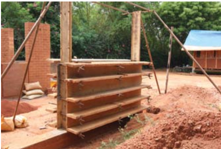
Formwork for the wall
