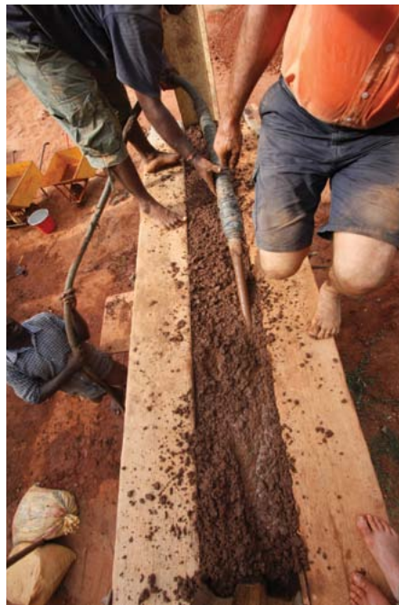
Vibrating the mix in the formwork
