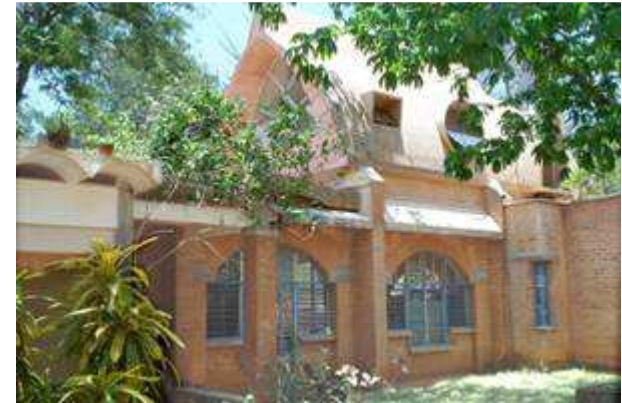
Office of the Auroville Earth Institute
