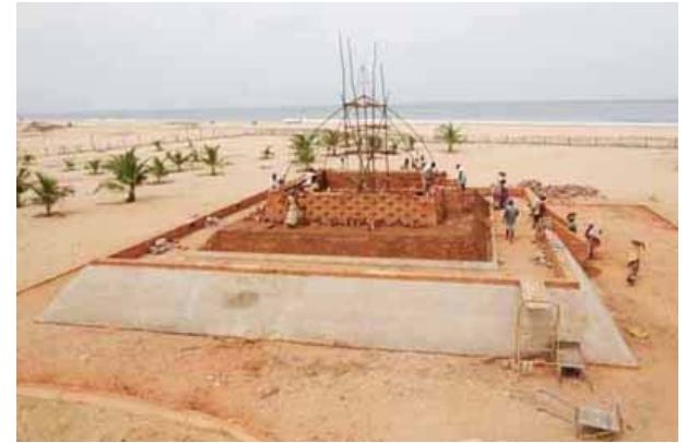
Dome and pyramid in progress
