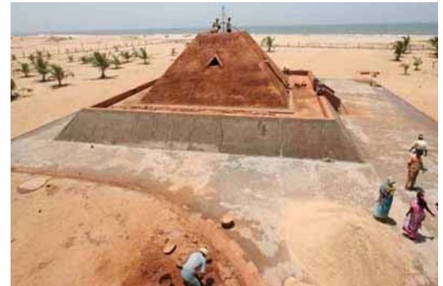
Completed dome and pyramid
