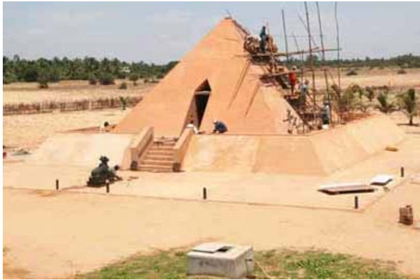
Cladding the pyramid with over stabilised blocks
