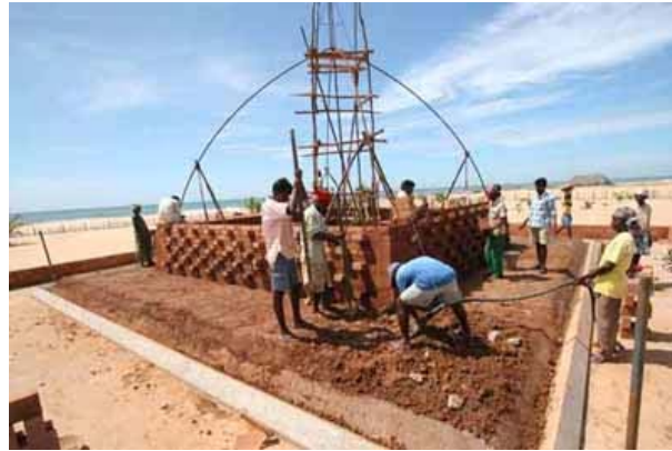
Filling the pyramid with a plain earth concrete
