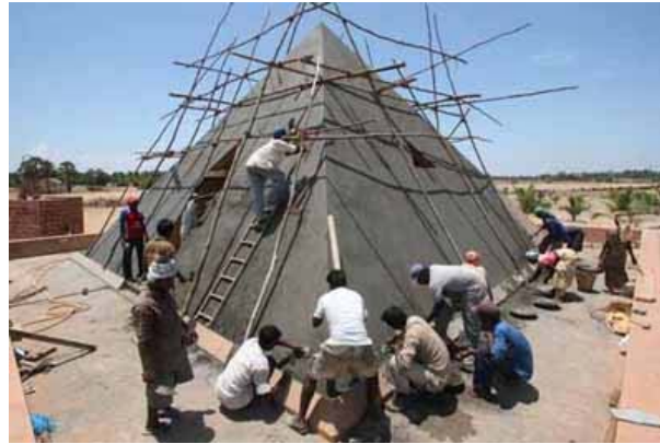
Waterproofing the pyramid with a cement sand plaster
