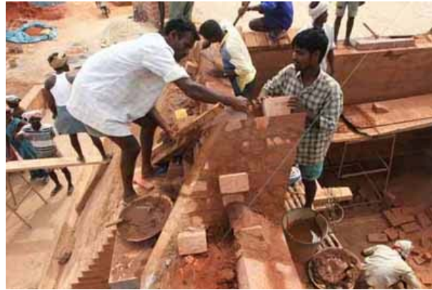
Building a triangular arch for the windows
