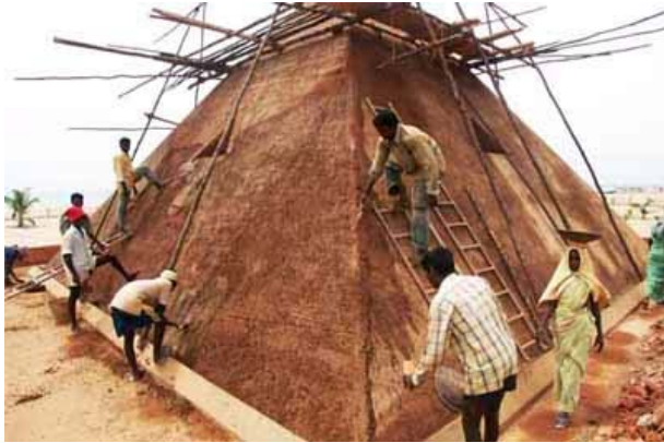
Plastering the pyramid with a thin layer of earth concrete
