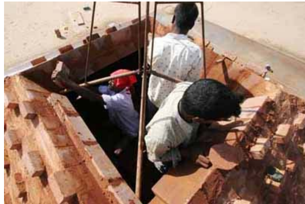
Bond pattern toward the end of the dome
