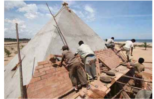
Cladding the pyramid with over stabilised blocks
