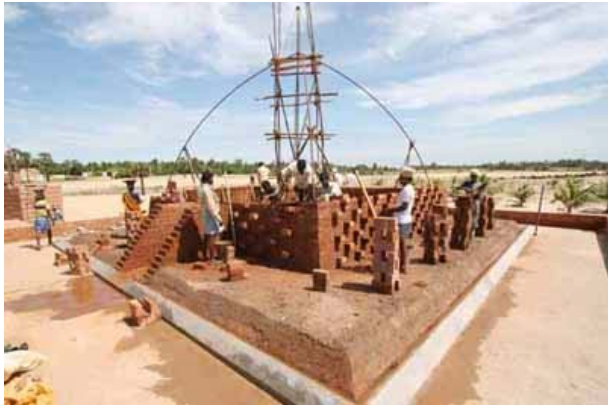
Keys of the dome, to be linked with the pyramid filling
