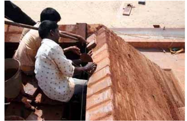
Bond pattern in the corner of the dome
