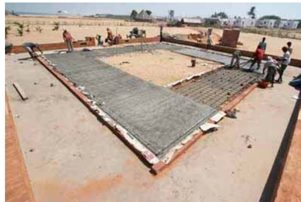
Casting the reinforced concrete slab of the pyramid
