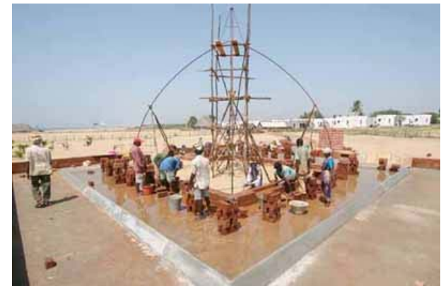
Starting the cloister dome with the template
