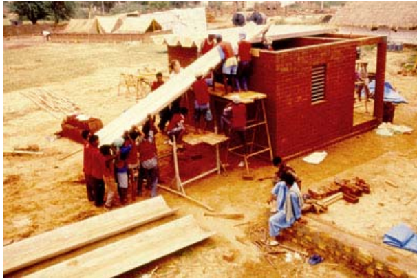
Aum house under construction – Lifting channels after 44 h
