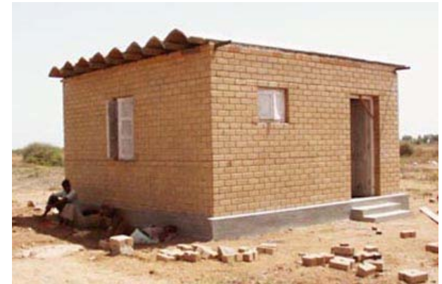
Model house with ferrocement channels
