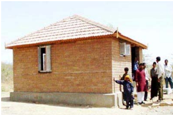
Model house with Mangalore tiles with 4 sides roof
