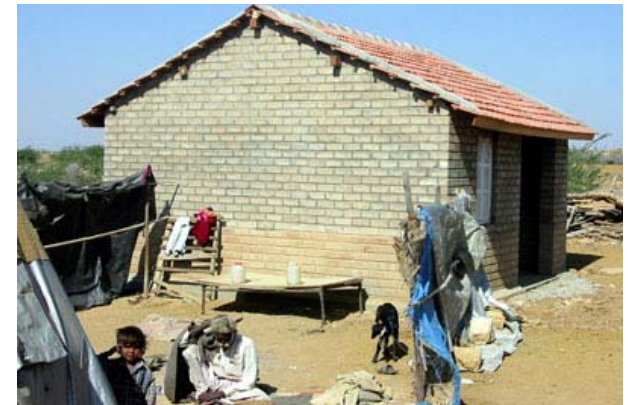
Model with Mangalore tiles with 2 sides roof
