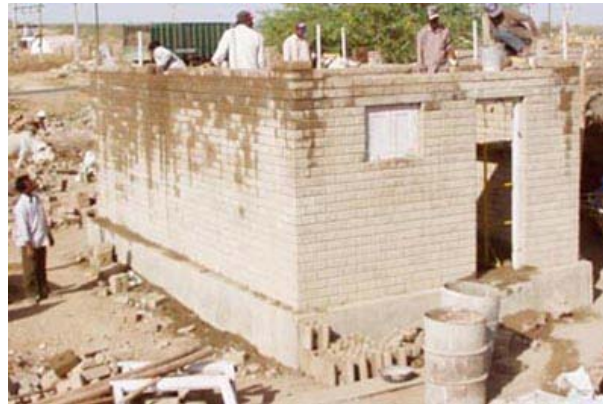
Training course for building a model house
