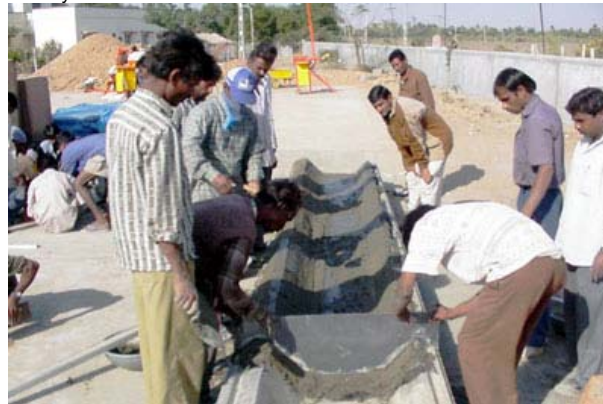
Precasting ferrocement channels
