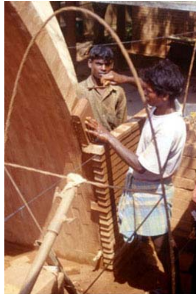
Building a Lunette with the Free Spanning technique
