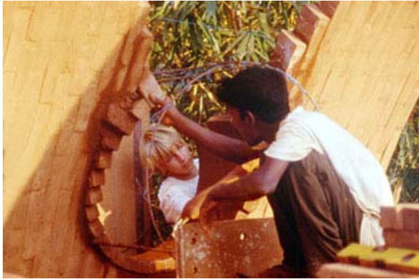
Building a bull eye with the Free Spanning technique
