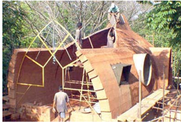
Building an equilateral vault with the free spanning technique
