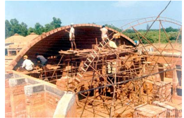
Building a 10.35 m span Segmental vault, with the free Spanning technique
