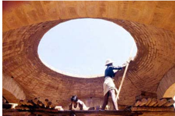
Building a hemispherical dome on pendentives
