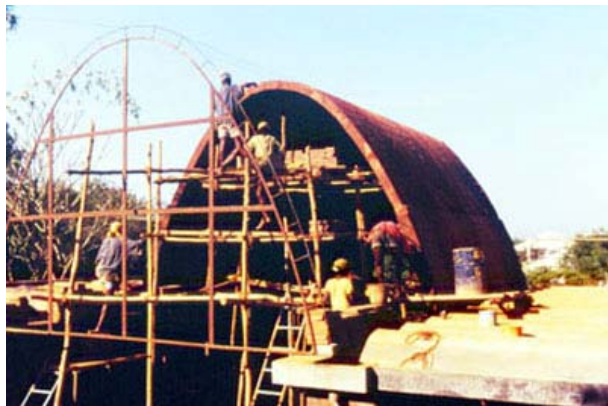
Building an Egyptian Vault with the Nubian technique
