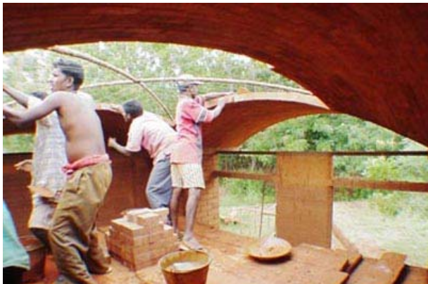
Building a groined dome with the Nubian technique
