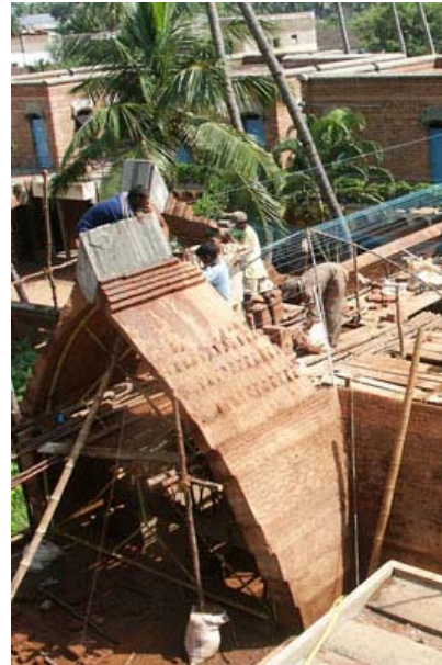
Building a equilateral groined vault at Pondicherry
