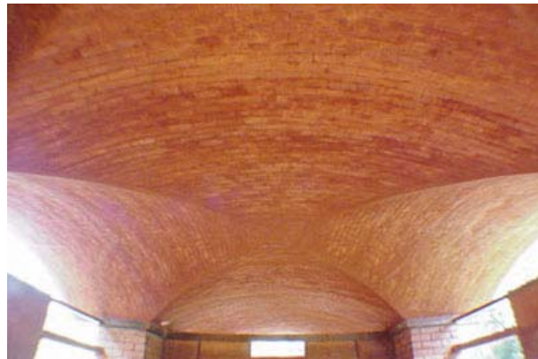
Groined dome and vault, 3.48 m span
