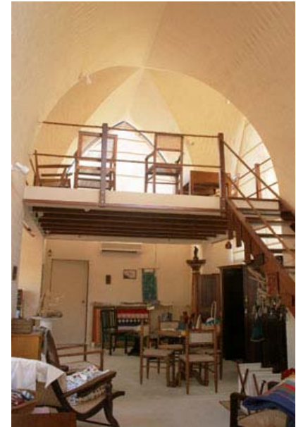
Equilateral groined vault at Pondicherry
