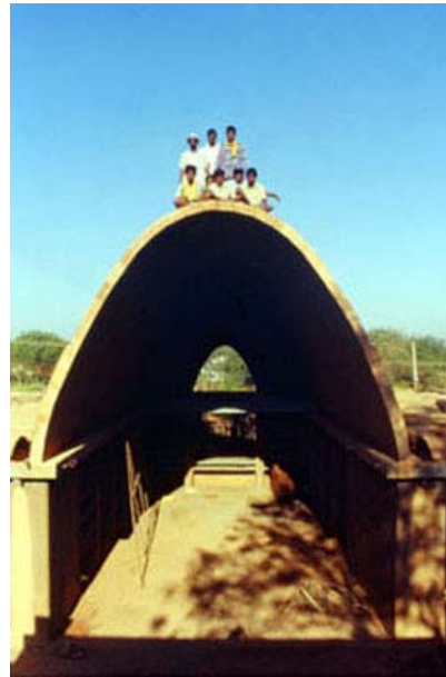
Egyptian Vault, 5 m span, 9 m long completed in 12 days with 4 masons
