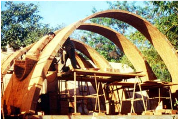
Building a catenary vault with the Nubian technique
