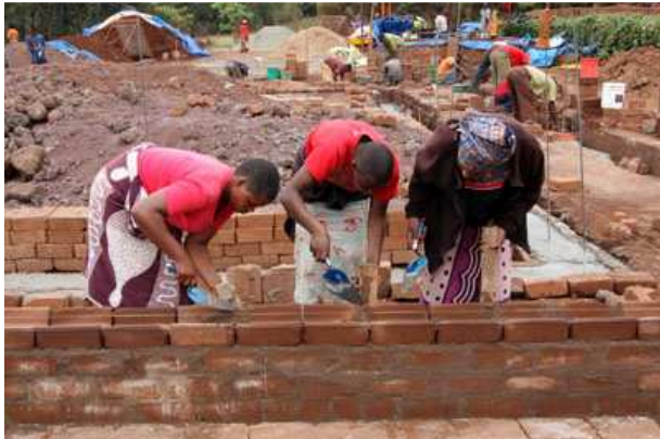
Ladies masons under training
