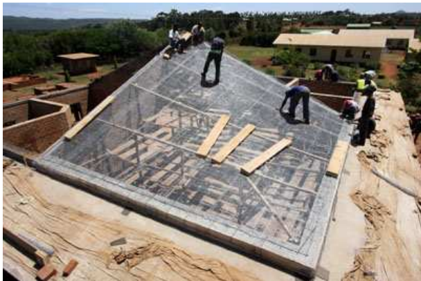
Laying the chicken mesh of the hyperbolic paraboloid roof
