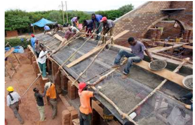
Casting the ferrocement of the veranda
