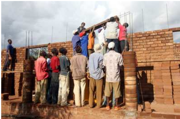
Laying the composite lintels
