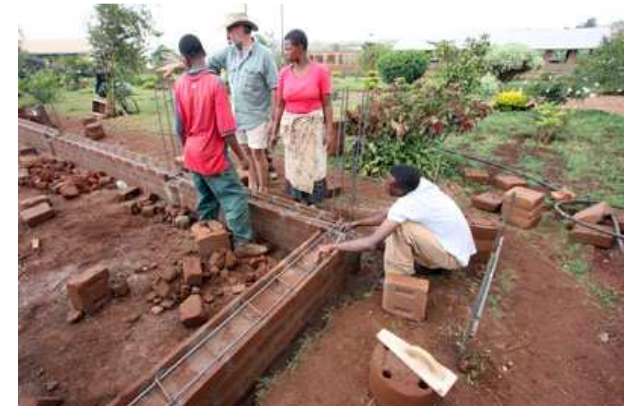
Eng. Douglas Ommanney supervising the plinth beam
