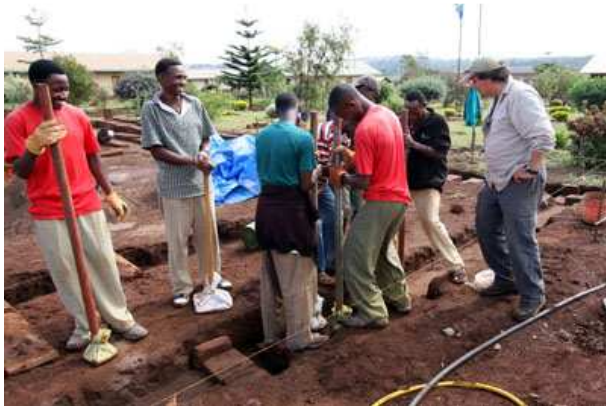
Mr. Alberto Navarro supervising the rammed earth foundations
