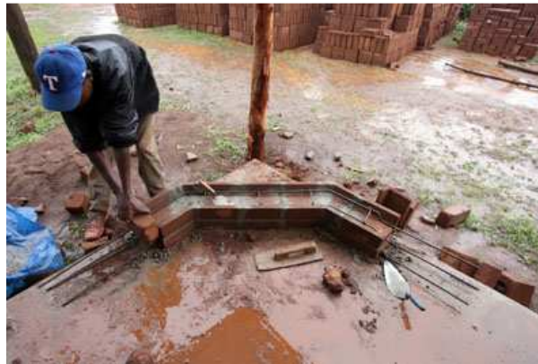
Precasting composite lintels
