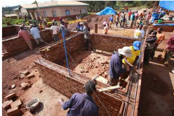
Preparing the composite beam of the sill
