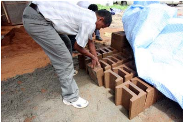
Initial stacking and curing of U blocks below plastic sheets
