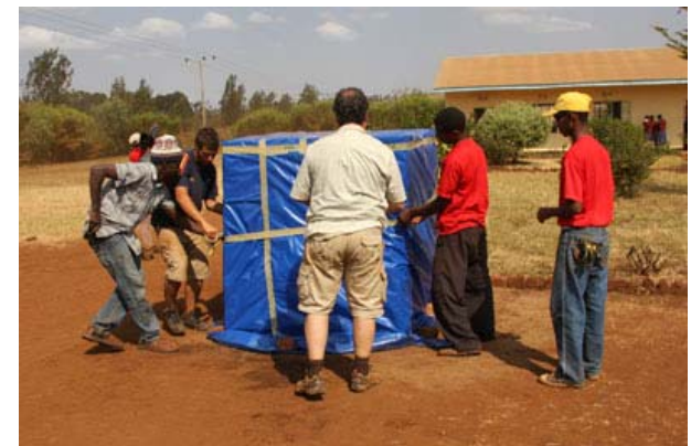
Final stacking of the block and curing below plastic sheets
