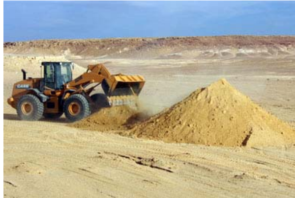
Mixing the selected veins of soils in the quarry
