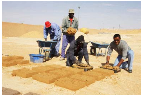
Mr. Ibrahim Bachir Malik moulding stabilised adobes
