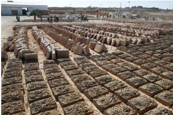
Mass production with 2 mixers and 3000 adobes per day
