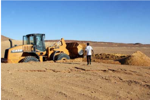
Doing some test pits to evaluate the soil quality
