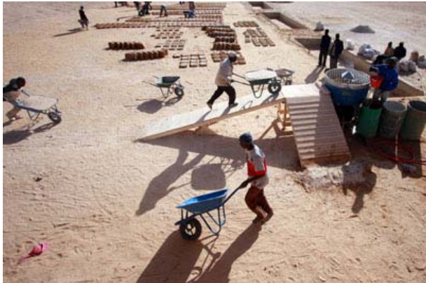
Optimised production of adobes with a mixer
