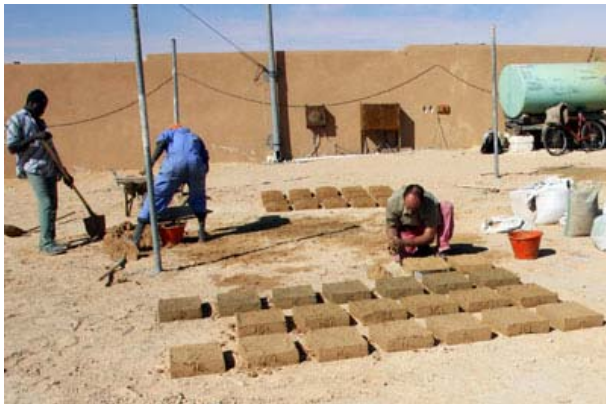
Moulding stabilised adobes with various stabilisers
