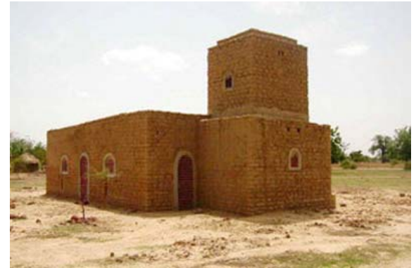
Top vault is just finished
