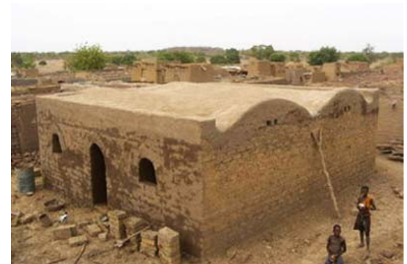
Completed vaulted roof
