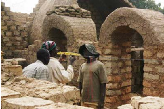
Setting-up and levelling of the guide cable
