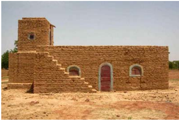
Flat terrace roof & infill between vaults and side walls
