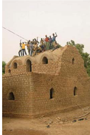
Topping out of 2 nd floor vault
