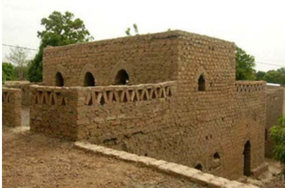
Completed 2 nd floor vault (flat roof) and terrace
