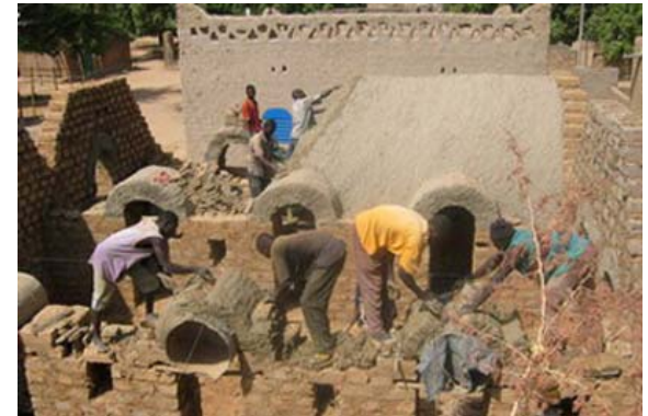
Construction of the vault
