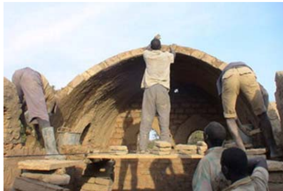
Construction of a nubian vault
