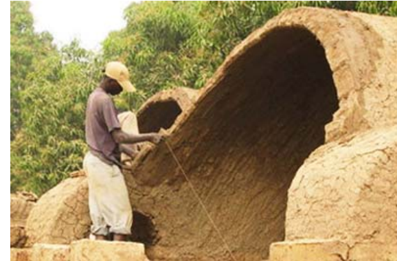
Vault construction using the compasses, which slides on the guide cable
