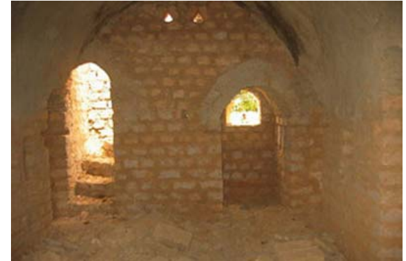
Internal view of the staircase
