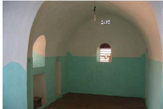
Interior with lime wash walls and cement floor
