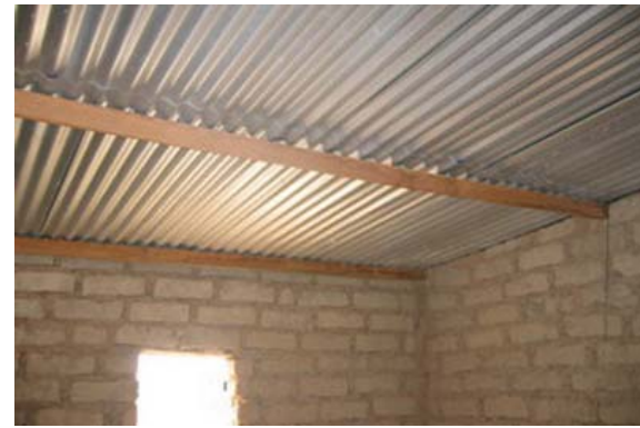
"Modern" roofing in the Sahel
