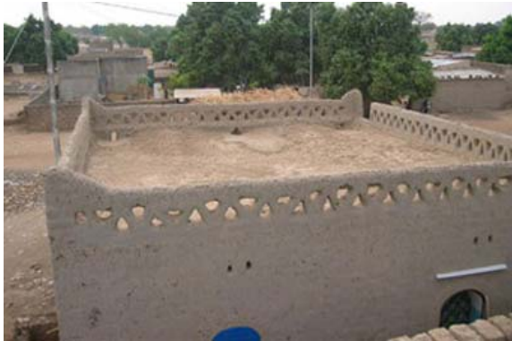
Flat terrace roof, with infill between vaults and side walls
