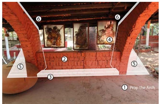
*Tilting arches at tree well requiring tie-back*
