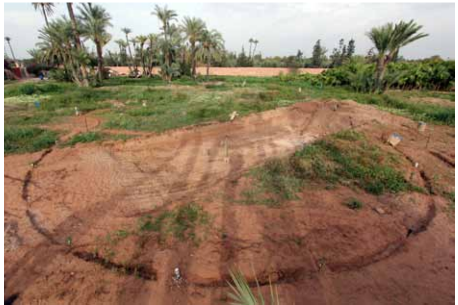
Marking the outline of the building on the site
