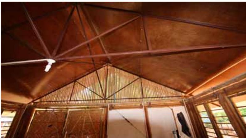
*Steel trusses & ply-wood ceiling*
