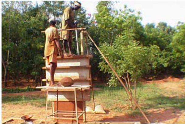
Rammed earth form 100, for doing walls of 36.5 to 99 cm & 240 cm high
