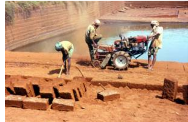
India, Orissa, Near Narangarh – Petroplinthite cutting
