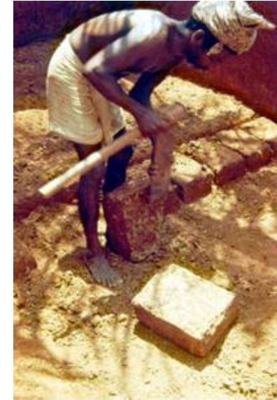
India, Kerala, Near Soranad – Shaping a plinthite block
