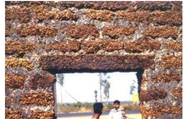
India, Orissa, Near Bhubaneswar – Lintel – 75 cm span
