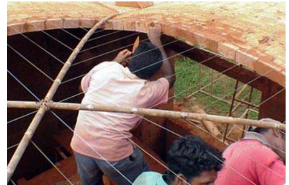
Starting the segmental groined dome
