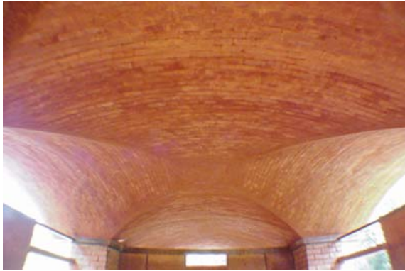
Segmental groined dome completed in 5 days with 4 masons
