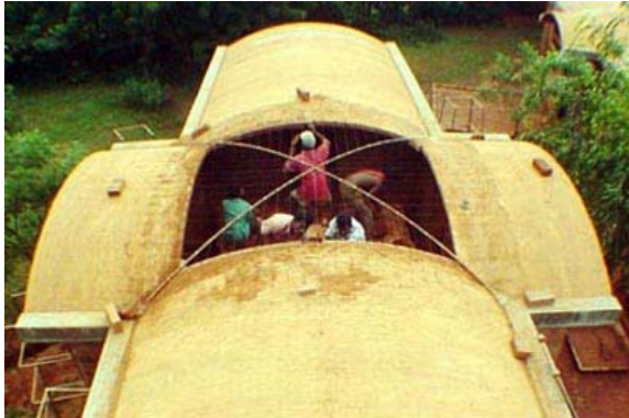
Building the segmental groined dome
