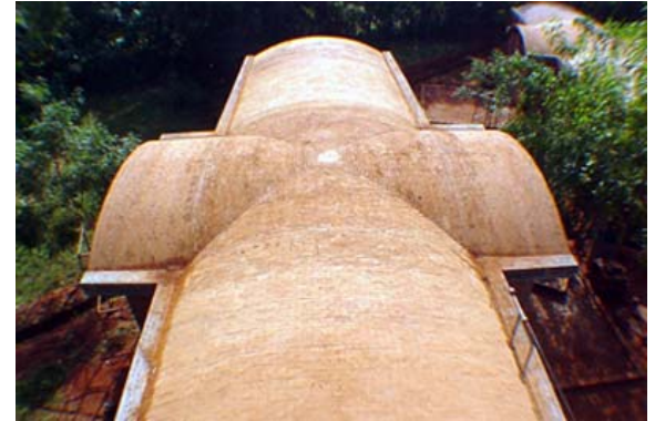
Segmental groined dome completed in 5 days
