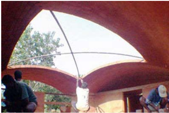
Laying blocks in the corner
