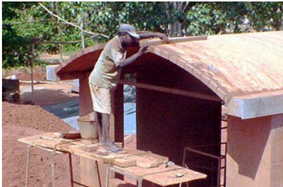
Completing the vault and controlling the shape with a straight edge
