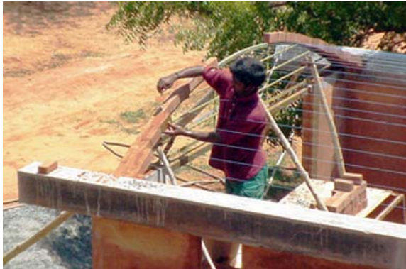
Building the segmental vault on the window frame as a template
