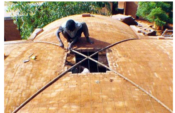
Groined dome towards completion
