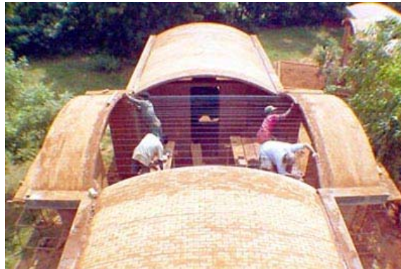
Building the side vaults
