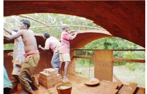
Building the segmental groined dome with 4 masons
