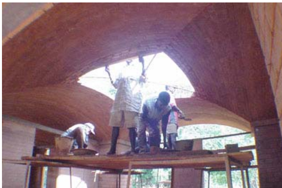
Completing the groined dome
