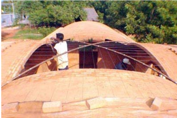
Building the segmental groined dome
