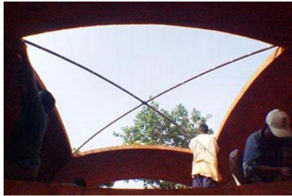
Segmental groined dome in progress
