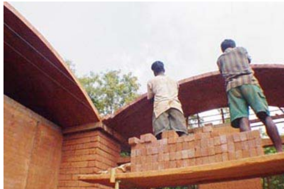
Finishing the side vault
