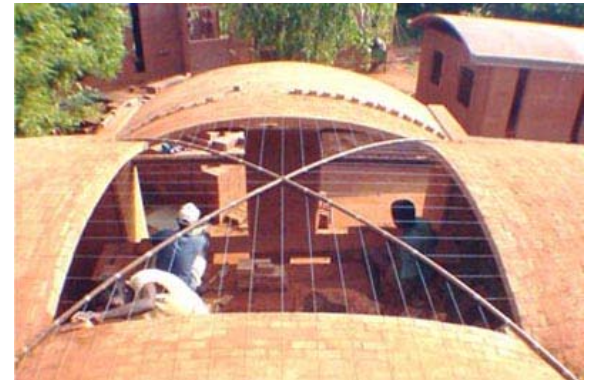
Fixing the steel template and starting the groined dome
