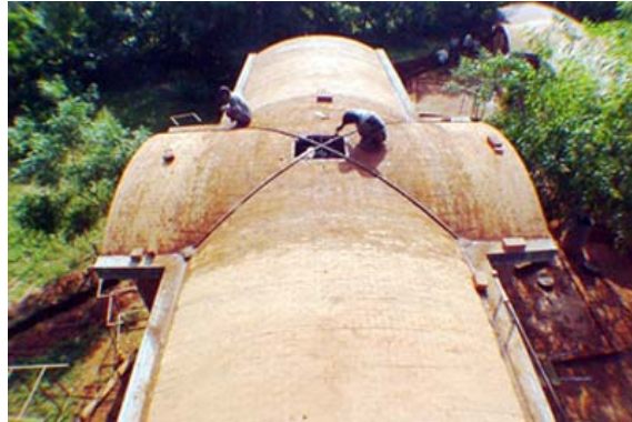
Segmental groined dome near completion
