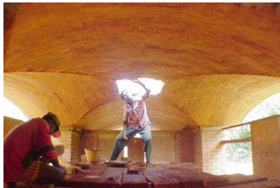
Finishing the dome with 1 mason
