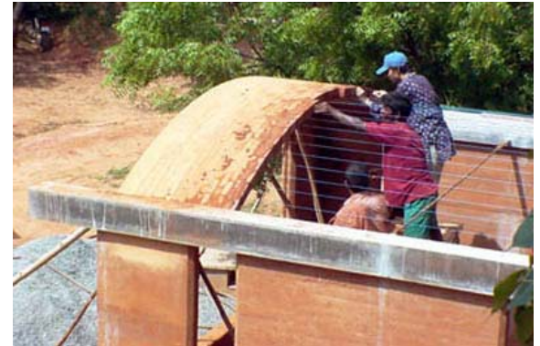
Building the segmental vault above the bedroom
