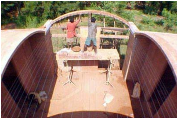
Starting the side vaults
