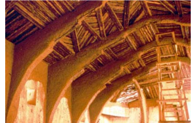
Nigeria - Reinforced earth - Photo CRATerre/ENSAG
