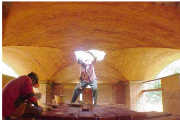
Finishing the dome with 1 mason
