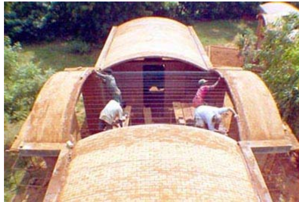
Building the side vaults
