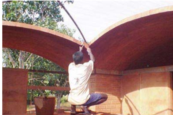
Adjusting a block in the corner of the groin
