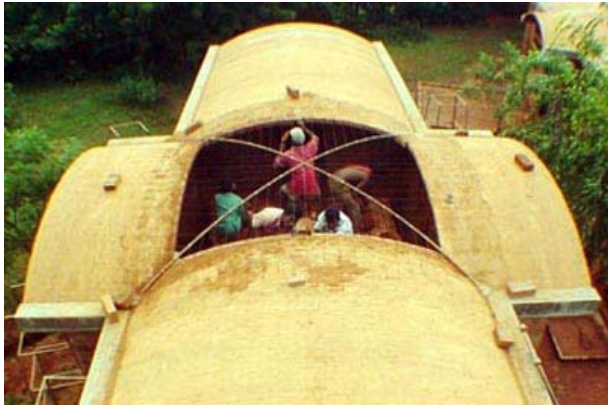
Building the segmental groined dome
