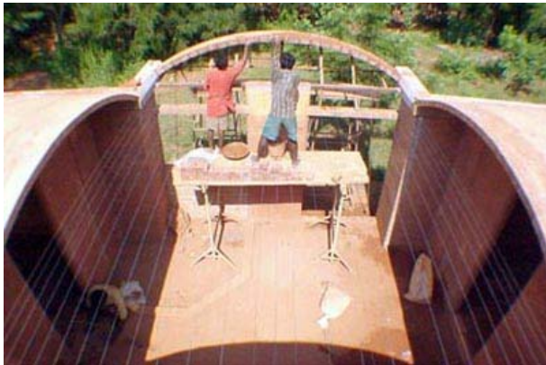
Starting the side vaults
