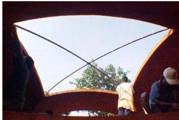
Segmental groined dome in progress
