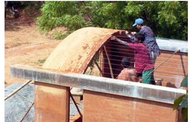
Building the segmental vault above the bedroom
