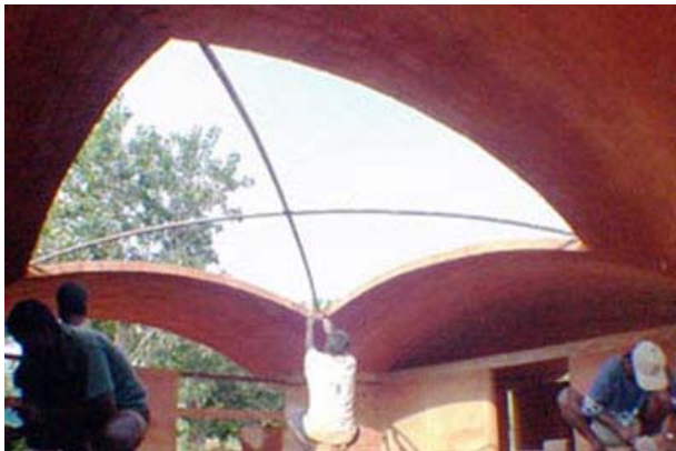
Laying blocks in the corner
