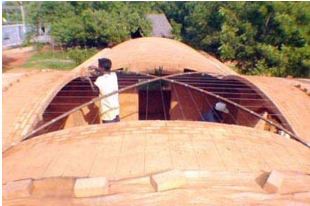
Building the segmental groined dome
