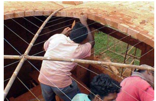
Starting the segmental groined dome
