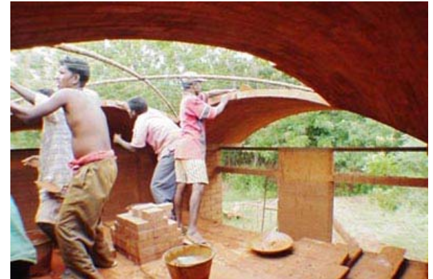
Building the segmental groined dome with 4 masons
