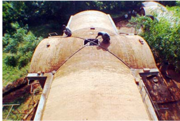
Segmental groined dome near completion
