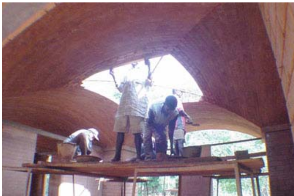
Completing the groined dome
