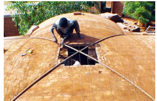
Groined dome towards completion
