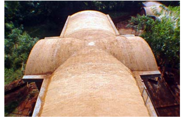
Segmental groined dome completed in 5 days
