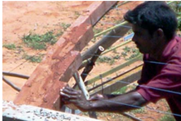
Building the segmental vault by steps to start with
