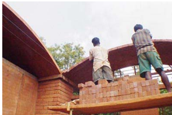
Finishing the side vault
