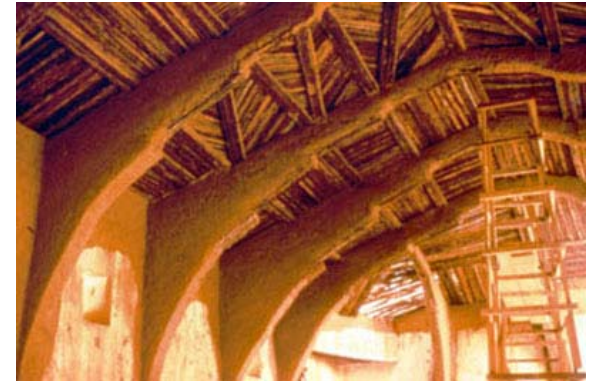
Nigeria - Reinforced earth - Photo CRATerre/ENSAG
