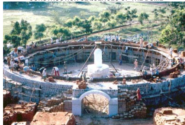
Granite vault completed and dome after 1 week
