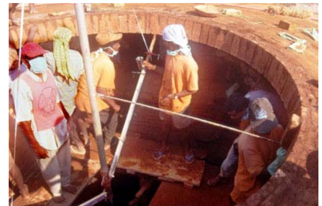
Dome near completion
