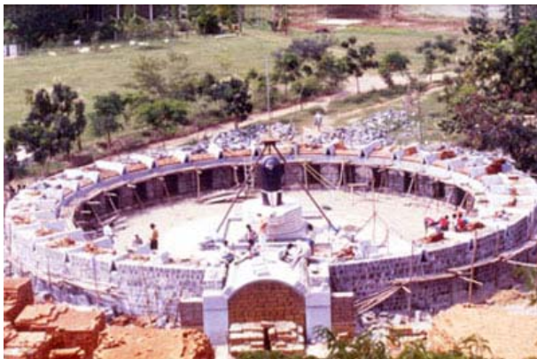
Starting the dome and the granite vault on the 21 st November 1998
