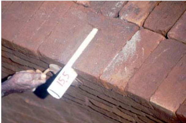
Inserting a pipe for an acoustic corrector to absorb 620 Hz
