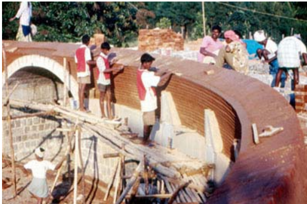
Plastering the parts of the course which are too low
