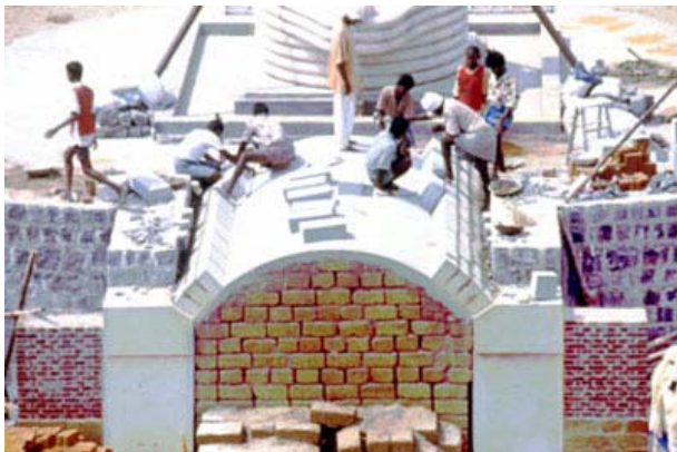
Starting the entrance vault with granite blocks
