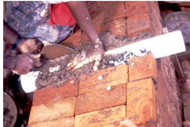
Inserting the pipe for an acoustic corrector to absorb 220 Hz
