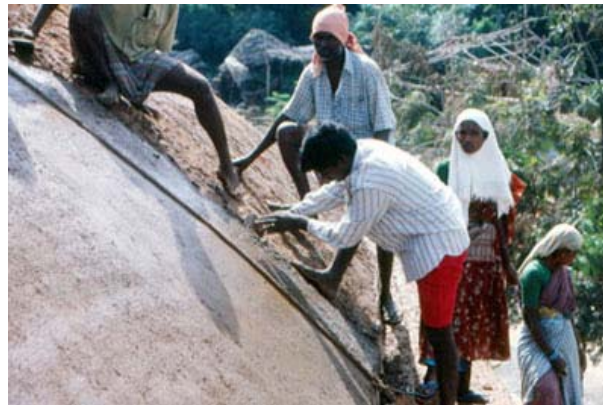
Smoothing the earth concrete with a stabilised earth plaster
