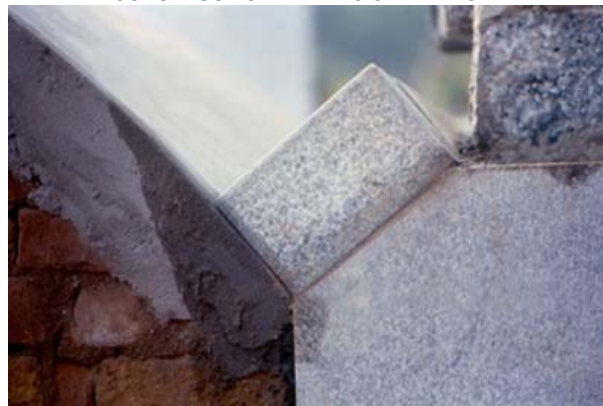
Block touching the springer at the intrados
