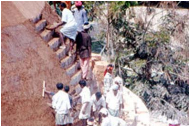
Smoothing the granite steps with an earth concrete
