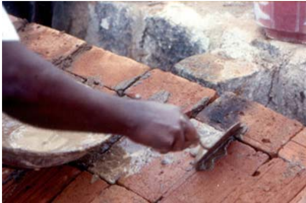
Grouting the stabilised earth glue in the joints
