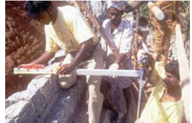
Loading the haunches with granite stones
