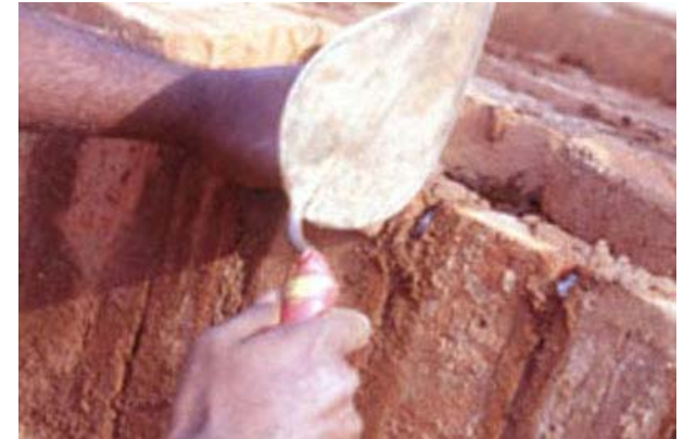
Starting the dome with 29 cm thick blocks
