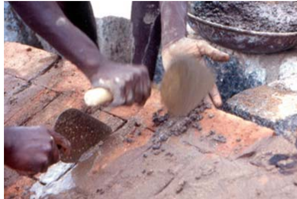
Filling tightly mortar with stone chips
