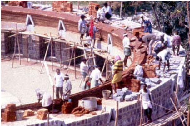
Beginning the dome
