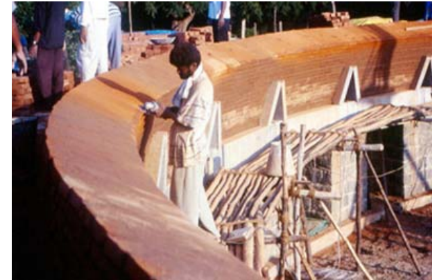
Grinding the parts of the course which are too high
