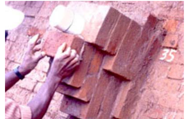
Closing the pipe of an acoustic corrector
