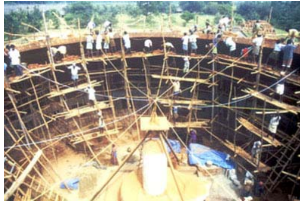
Working with an average of 25 masons
