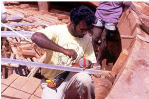
Adjusting the compass for the upper courses
