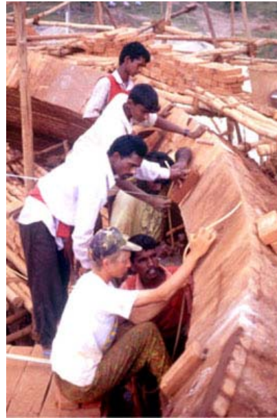
Checking the level of the courses
