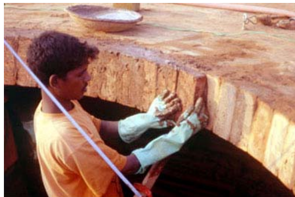
Laying the last courses, 21 cm thick
