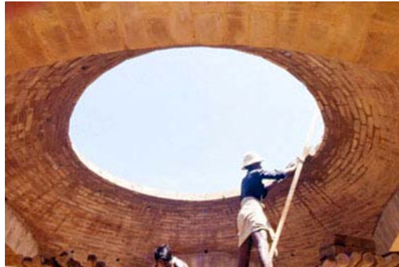
Building a dome on pendentives, 3.70m span
