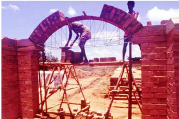
Building a segmental arch, 2.38m span
