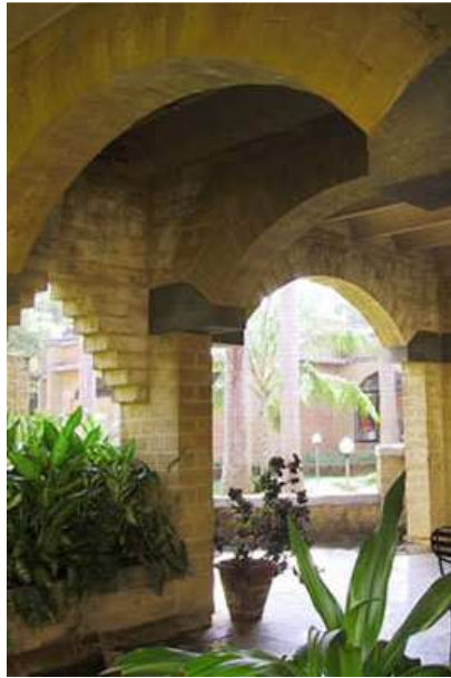
Gallery towards the courtyard
