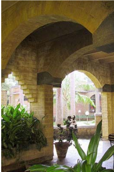
Gallery towards the courtyard
