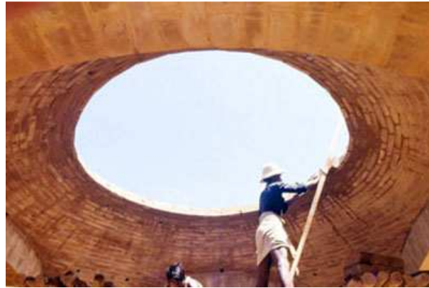
Building a dome on pendentives, 3.70m span
