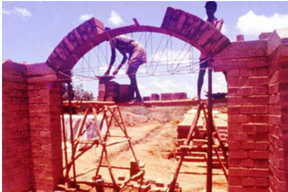
Building a segmental arch, 2.38m span
