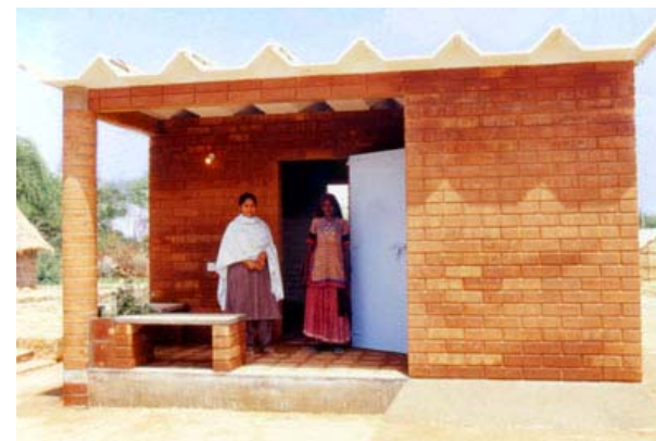
Aum House at Khavda, Gujarat, India – 2001
