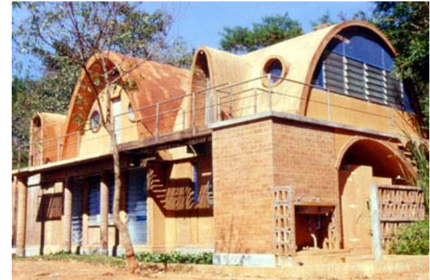
Training centre of the Auroville Earth Institute
