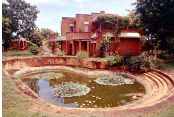
Quarry used for a biological wastewater treatment (lagooning)
