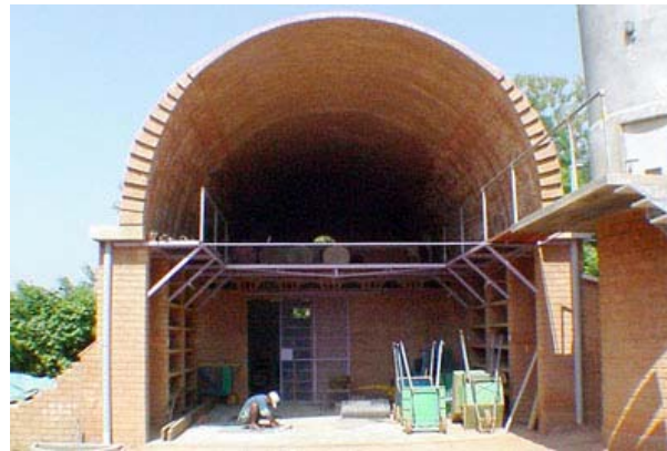
Semicircular vault, 6 m span built free spanning in 6 weeks
