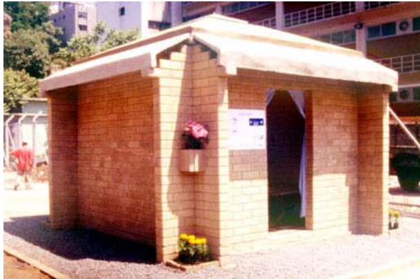
Minimum emergency house built at Istanbul, Turkey, in 8 days During the City Summit habitat in 1996
