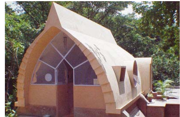
Equilateral vault, 3.6 m span built free spanning in 6 weeks
