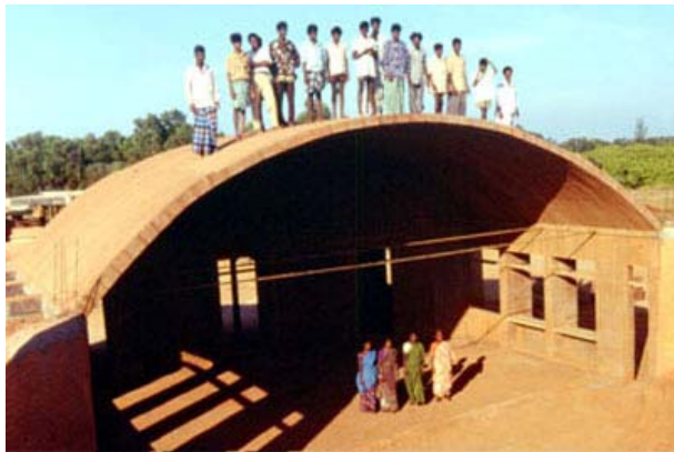
Segmental vault, 10.35 m span built free spanning in 3 weeks
