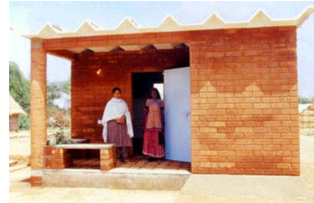
Aum House built in 62 hours in Gujarat For the rehabilitation after the 2001 earthquake
