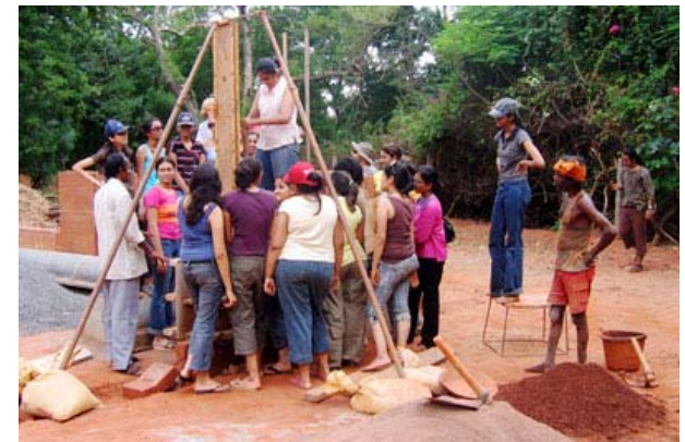
Awareness programme on stabilised rammed earth walls
