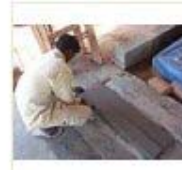
05 Precasting various pieces
