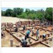
06 Doing the basement
