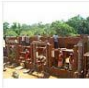
07 Building the first floor
