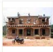
08 Building the second floor
