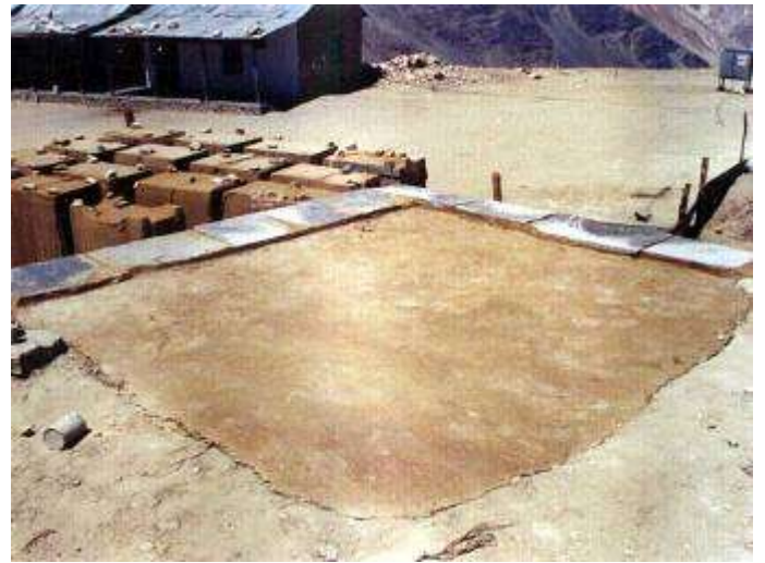
Roof in progress with stone slabs on the sides
