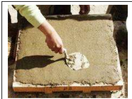
11. Smoothing the last coat with a trowel
