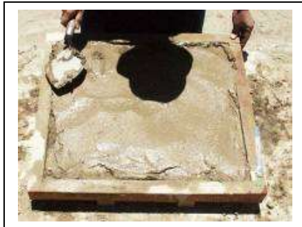
8. Applying the 4 th coat
