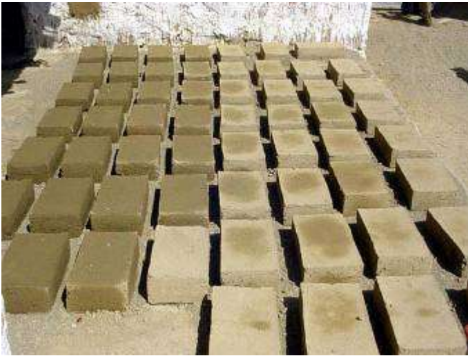
Moulding of new adobes
