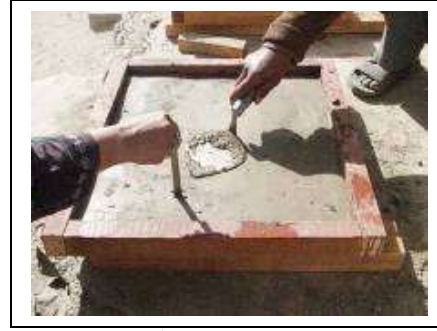
3. Applying 2 nd coat & checking thickness
