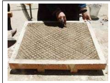
9. Scraping the coat and soaking it after
