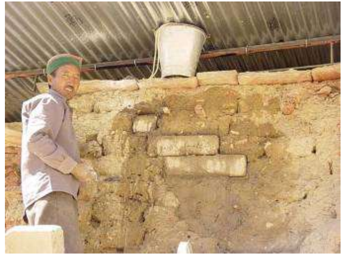
Repairing walls with new adobes
