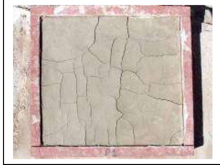
5. Cracks of the 3 rd course with Tua clay
