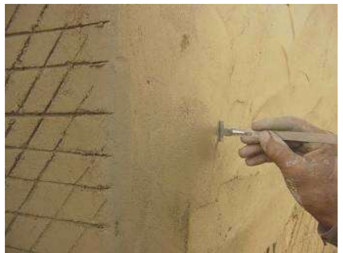
Checking the thickness of the earth plaster
