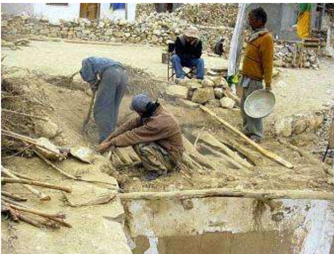
Removing the old roof
