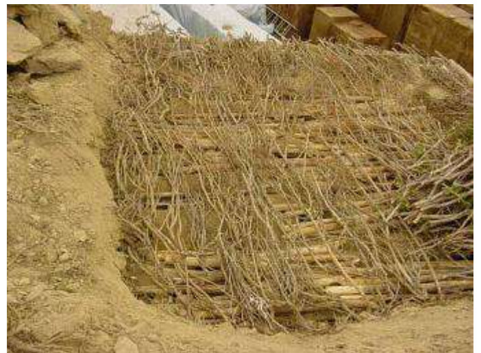
Laying the new scrubs for the roof
