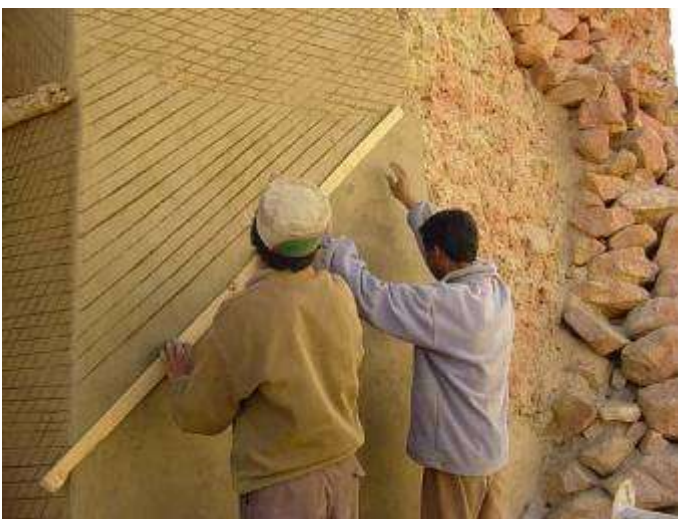
Plastering walls with earth mixes
