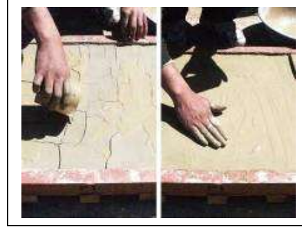
6. Filling cracks of the Tua course
