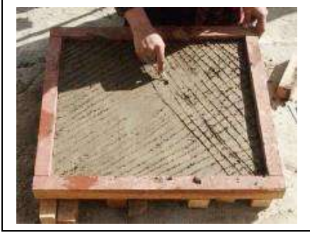
4. Scraping every coat before the next one
