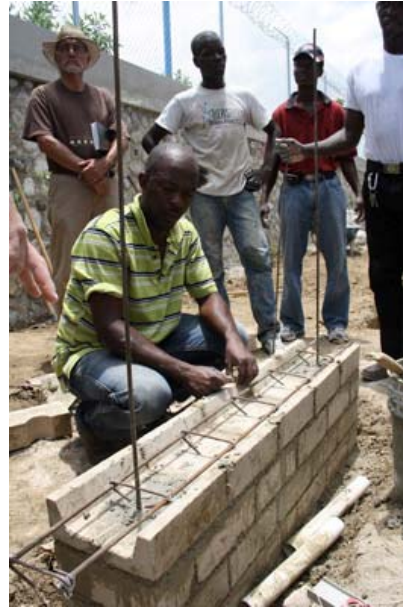
8. Reinforcement of the plinth beam
