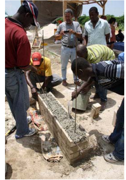
9. Casting concrete of the plinth beam
