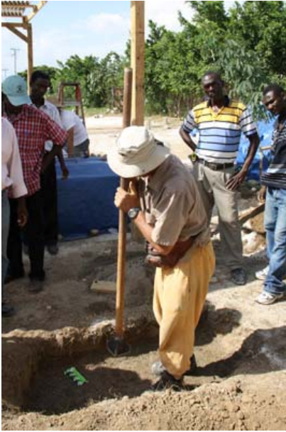
7. Ramming a stabilised reamed earth foundation
